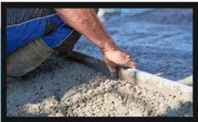
Plaster & Screed Concrete
