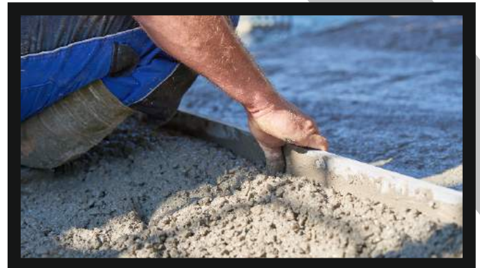
Plaster & Screed Concrete
